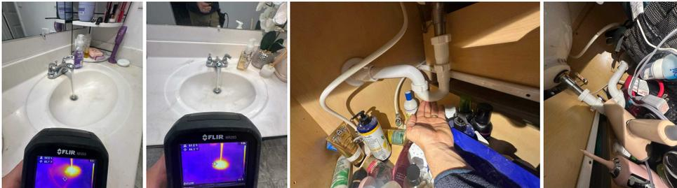
32. Acceptable Faucets/Traps: Delta fixtures with a metal trap
