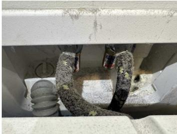
9. Marginal Dryer Vent: Metal flex - The laundry vent appears to be dirty and may need cleaning. Recommend having it cleaned to ensure proper ventilation and prevent potential hazards
