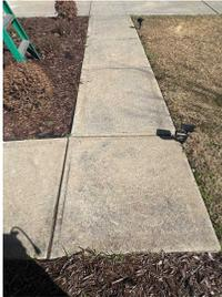
3. Acceptable Patio: Concrete - A minimal crack was observed on concrete patio floor. This appears to be a minor cosmetic issue with no immediate concerns. Monitoring for any changes over time is recommended.
