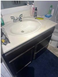
8. Acceptable Faucets/Traps: Delta fixtures with a metal trap
